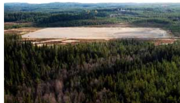
Bofors Test Center has an optically registrable surface measuring 300 x 300 m that is also a take-off and landing runway.
